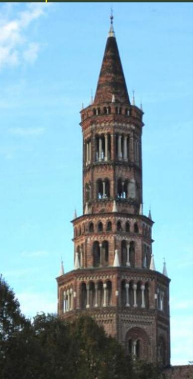
The bell tower, octagonal in plan, rises starting from the tiburium and consists of two sections, a first 4.14 meters high and a second of 12.19 meters, from which finally the terminal conical section starts, resulting in a total of 56.2 meters.
