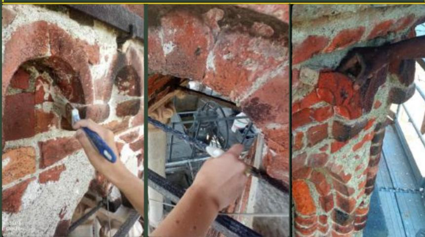
For the restoration were used mortars BioCalce Pietra®, Geocalce® F Antiseismic and GeoCalce® FL Antiseismic of the brand Kerakoll SpA (evaluated with the highest level of GBR) which contain only raw materials of natural origin and recycled minerals, have a reduced environmental impact in their emissions of CO<sub>2</sub> and volatile organic compounds (VOCs) and are recyclable as inert at the end of their life cycle.
